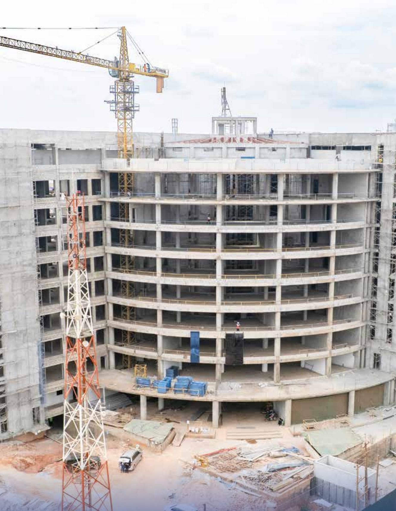
Aerial view of the UETCL new head office building under construction.
