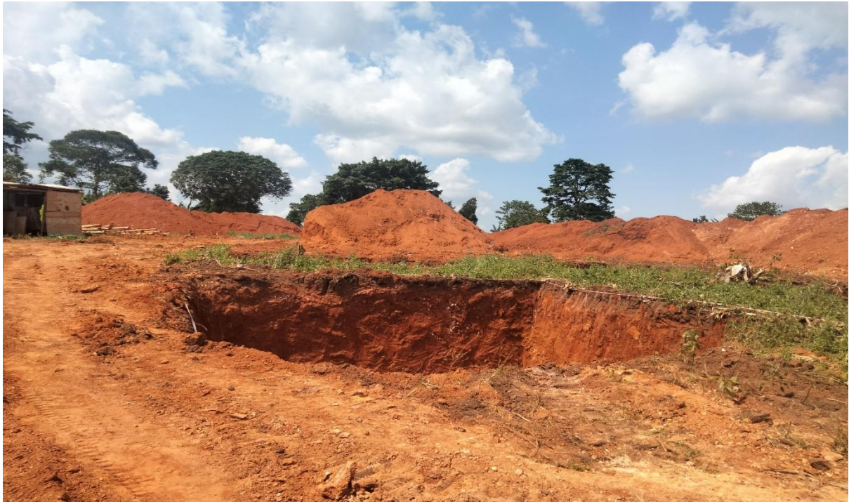
Picture 3: Excavation of tower bases on going
