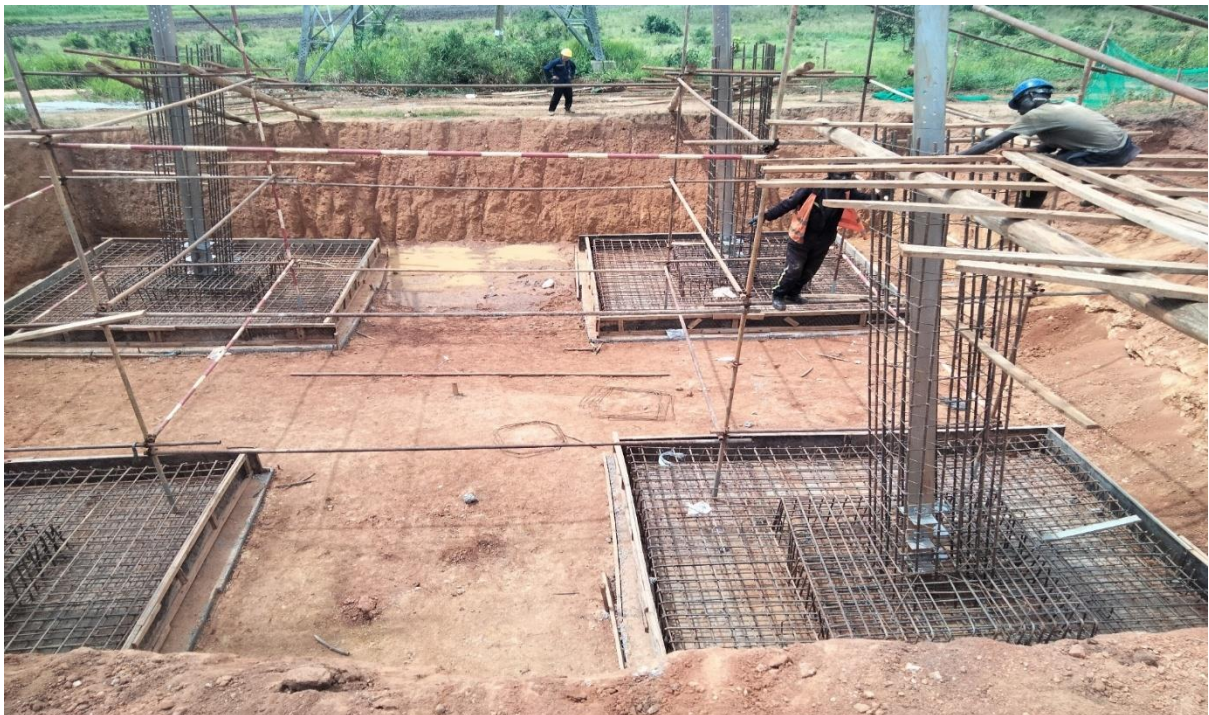
Picture 4: Construction of a Tower base is ongoing (Steel works)
