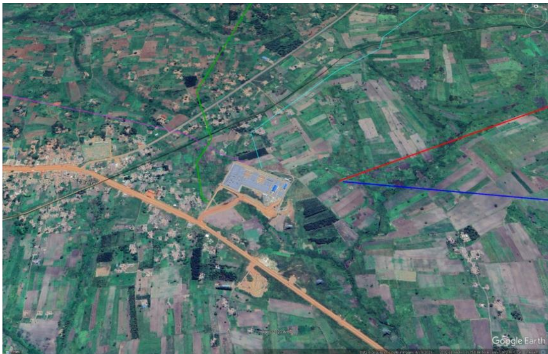
Figure 4-4 – Location of Olwiyo substation; existing 132 kV transmission lines are marked in cyan (Olwiyo – Gulu) and magenta (Olwiyo – Nebbi).
