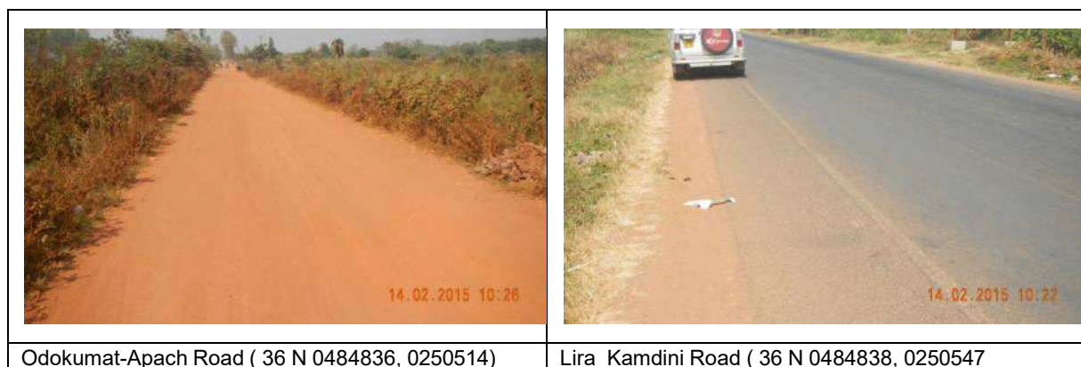
Picture 6-10 Types of Road in the Project Area – Lira District
