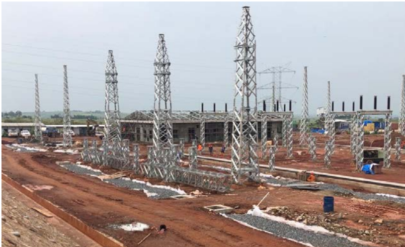
Ongoing works at 132kV Olwiyo substation
